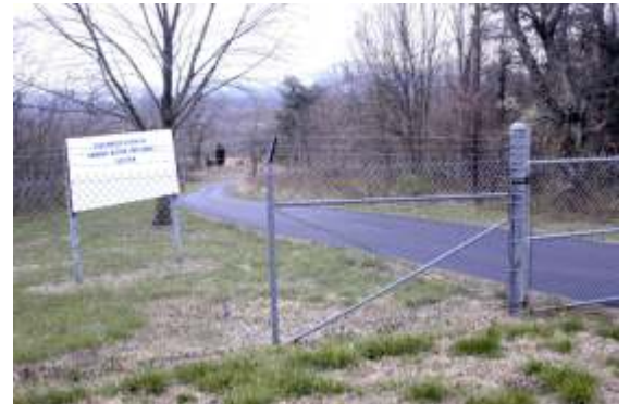
(Top) Fenced entrance to Superfund site. (Bottom) Abandoned Greenwood School building.
