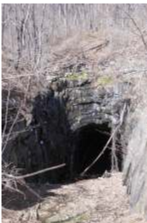
East portal of original tunnel.
